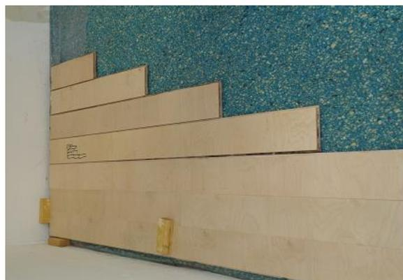
Cut the Lumaflex panels in order to obtain an homogeneous resistance before assembling. Minimum panels length : 790mm.
