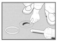
Around flush drain openings, heat the sheet and mark the location of the drain using a clamp ring. Then cut a small hole in the centre of the drain within the mark. Heat the flooring and press the clamp ring down into the edge of the drain. When using an adjustable clamp ring, make sure it fits tightly. Trim the material around the perimeter of the ring. Alternatively; use cutting tool as per recommendation from the drain manufacturer.
