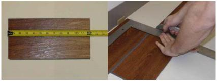
5. The remaining piece cut from the last plank in the first row may serve as the first plank in the second row provided it is at least 30 cm long. Always cut end joints from row to row a minimum of 30 cm.
