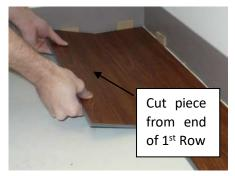
6. Install the long side of the first plank of the second row. Remember to place a 6 mm or 12 mm spacer between the wall and the short side of the plank. Insert the tongue side into the groove side of the previous row at a natural angle and rotate downward until plank is flat with the substrate. You should only have to lift the plank high enough to get your fingers underneath to achieve this natural angle
