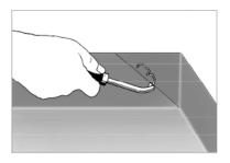
All seams on floor and coving must be grooved before welding.
