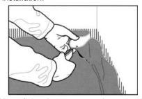
When fitting in-corners, make a cut in the excess material starting about 5 mm (about ¼ in.) above the floor in the corner. If the material has to be heated before folding, heat the area between the sheet and the wall. This provides better contact between the sheet and adhesive.
