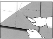
When fitting an out-corner, the sheet is folded against the corner and cut about 5 mm( <sup>1</sup>/<sub>4</sub> in.) from the floor. The guidelines in the picture show the corner on the sheet and the position of the cut at about a 45degree angle. Then a diagonal cut is made as shown.
