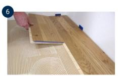
Repeat steps 2-4, pick up and spread glue. Start the second row of boards with the cutoff board from the first row. Get the floor board into place in the groove track and press it down into the glue.
