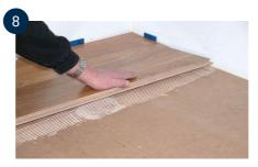
Go back along the board row while pressing the row down against the subflooring (into the glue). Proceed as described in points 6-8.
