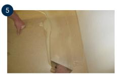
Pick up the board row that has been laid out. Spread glue on the subflooring, corresponding to the entire row of boards. Lay the floor board by board, and put a wedge against the wall.
