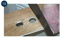
Saw off the piece to be placed behind the pipes, closest to the wall. Saw at an angle as shown in the picture. If the holes are located on the short end of the board, the board is cut at a 90° angle straight through the holes. Spread MS adhesive on the subflooring and then wood adhesive on the sides of the board that is to be fitted. Knock the board into place and cover with pipe collars.
