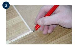
With a pencil, mark the cut 4-5 mm from the short end of the previous board to make it easier to lower the board into place.
