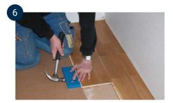
Lay the floor board by board, and put a wedge against the wall. Repeat steps 1-5, starting with the cut-off board. Note that there should be at least 500 mm between end joints across the entire floor. This does not apply to start & stop boards.
