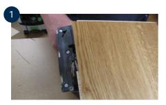
Before installing the first row, the protruding wooden profile on the board's tongue side must first be cut off.
