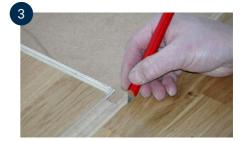
At the end of the row, turn the last board so that groove is against groove. Push the short end tight against the wall. With a pencil, mark the cut 4-5 mm from the short end of the previous board to make it easier to lower the board into place.
