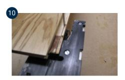
If there is no space to fold down the last board, it can be pushed in from the side instead. To do this, the tongue on the penultimate board row must first be straightened. Use e.g. a jigsaw or chisel and remove the protruding part at the end of the tongue.
