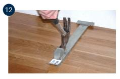
Spread out glue, lay down the last row of boards, and knock them in place using the percussion iron.
