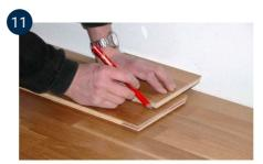
The last row of boards usually needs to be cut lengthwise. Lay the last board with the tongue against the wall, straight across and edge to edge with the penultimate row of boards. Add a piece of scrap board and measure the distance by sliding the board along the wall, while at the same time marking with a pencil where you need to saw the last board.
