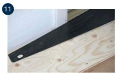
Door linings can be removed and moved up, but it is usually easier to saw them off. Use a loose floor board as a height template, and saw the lining with a fine toothed saw. Slide the floor under the liner. Also see point 10.
