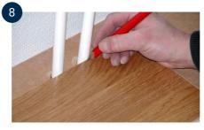
When there's a pipe at the long side of the board: - and how far from the edge of the board drill holes with a diameter of approx. 10 mm larger than the pipe itself. Measure how far from the end of the board the holes should be drilled
