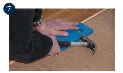
Always use Tarkett's tapping block, and never use a cut-off piece of board when joining the boards together.
