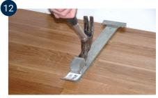
Spread out glue, lay down the last row of boards, and knock them in place using the percussion iron. Wedge against wall.
