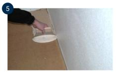
Pick up the board row that has been laid out. Spread glue on the subflooring, corresponding to the entire row of boards.
