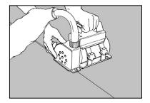
The sheets are heat welded. Do not weld until the adhesive has bonded completely. The joints are chamfered through the wear layer using a hand grooving tool or machine prior to welding. Groove 2/3 of the thickness for compact, till foam for acoustic.
