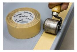
5. Remove the release liner from the remaining side of the PowerTape as well as from the back of the grit tape or Photoluminescent tape. Place the grit or Photoluminescent tape into the channel by starting at one side and working towards the opposite, ensuring that the 1/16" gap is equally maintained at both stringers.
