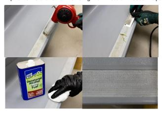
Cut new grit or Photoluminescent tape. Keep the grit or Photoluminescent tape back 1/16" from the stringer on both sides of the stair tread.
