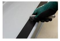
Starting at the cut in the strip using a metal scraper or chisel, lift the insert off of the tread and pull the Rubber Insert towards the stringer and away from the tread. Repeat the process for the other half of the strip.
