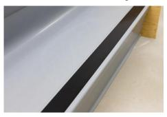
5. Cut a length of the 2" Tarkett PowerTape™ to match the length of the stair tread. Adhere it into the channel. Roll the tape with a hand roller to ensure bond.
