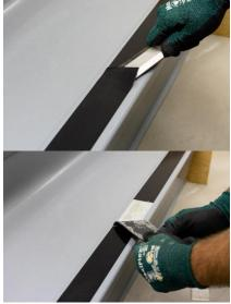
3. Remove all adhesive tape residue from the channel. Use a heat gun to soften the tape and scrape with a metal scraper or chisel. Denatured alcohol can be liberally applied to the channel to assist in the removal of the tape residue after scraping. (Follow manufacturer's precautions when using denatured alcohol.) NOTE: The adhesive residue must be completely removed prior to installation of the new Rubber Insert.
