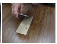
Using a straight edge and sharp utility knife cut completely through the plank along the lines. Using a hot air gun to warm the plank will make it easier to cut through the plank. Remove the center of the damaged plank.
