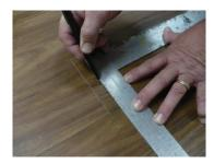
Mark lines on the plank to be replaced approximately one inch from the edges of the adjoining planks.
