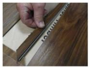
Carefully cut back from the corners of the plank at a 45° angle to the inside edges. Remove the edges of the cut plank. Do not distort or damage adjoining planks.
