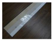
Position Tarkett S875 Floating Seam Tape so it is centered under the long side of each adjoining plank.
