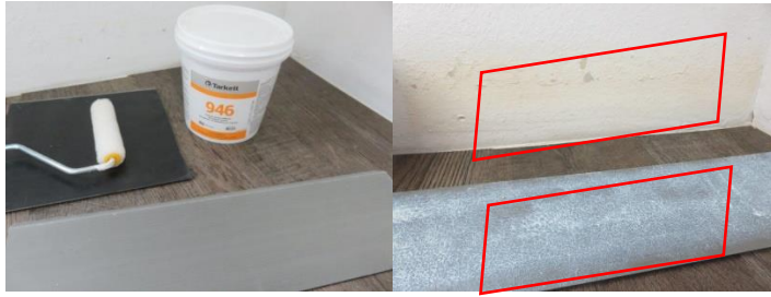
946 Applied evenly to both wall surface and wall base
