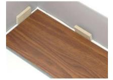
3. The end joints of the planks in the first row are assembled by inserting the tongue side into the groove side of the previous plank at a **natural angle**. Gradually lower the plank down flat until the end joint closes, insuring that the planks are perfectly aligned. Install remaining full planks in the first row.
