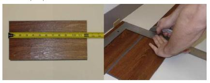
5. The remaining piece cut from the last plank in the first row may serve as the first plank in the second row provided it is at least 12" (30.4 cm) long. Always stagger end joints from row to row a minimum of 12" (30.4 cm).
