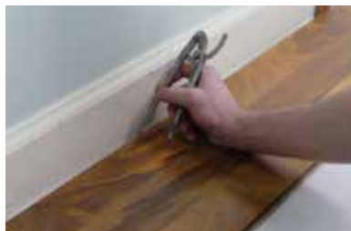
10. Scribe and cut first row, if starting wall is irregular.
