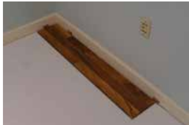
4. Begin laying planks left to right with tongue side against starting wall.
