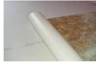
3. Install foam underlayment (Except Worthington). When installing over concrete, install an approved vapor retarder prior to installing foam underlayment.
