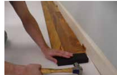
6. Using hammer and tapping block, gently tap along the groove side to engage each plank in first row. Tap in center of block. Continue in this manner to complete first row.
