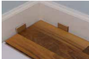
5. Place 5/16" spacers between wall and flooring. Align remaining planks in first row.
