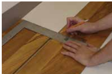
7. Measure and cut last plank in the first row. Allow for 5/16" spacer. Use a pull bar to engage last plank.
