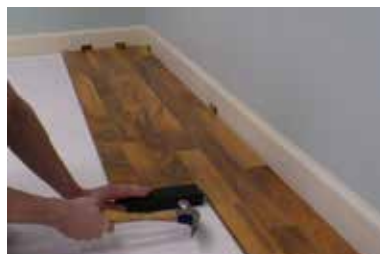
14. Using a hammer and tapping block, gently tap along the groove side to engage planks. Tap center of block.
