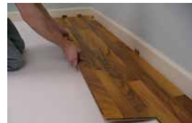
12. Install second plank by inserting the long side tongue at a low angle into groove side of previous row. Always stagger end joints from row to row a minimum of 12" (30.4cm).
