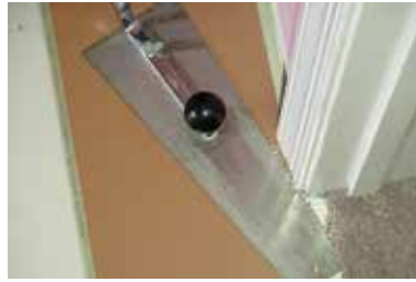
2. Undercut door moldings and casings.
