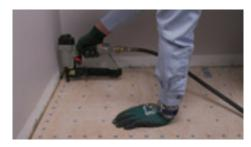
All wood substrates shall be double construction with the top layer being APA approved underlayment grade plywood, do not install directly over OSB, chip board, or luan.
