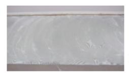
Apply QBond One adhesive using a 1/16"x 1/16"x 1/16" square notch trowel. Only apply enough adhesive that can be covered within 1-hour from the dry to touch state.
