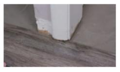
Undercut doorway moldings the thickness of the flooring.
