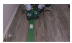
Measure and cut border piece. Border piece shall be no less than 2".
