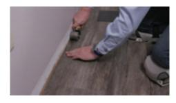
Install and roll with a small hand or J-type roller.
