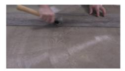
Install the first plank along the control line, paying particular attention to placement. Roll the leading edge with a small hand roller ensuring bond.
