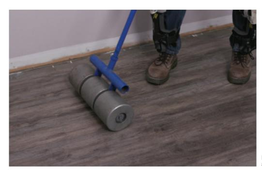
Roll flooring in both directions with a 75-100 lb. three section roller.
