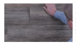
When installing planks in the adjacent rows hold plank at a 45 degree angle and slide horizontally until the plank engages. Pay particular attention to the stagger of the short end joints, the stagger shall be no less than the width of the plank in adjacent rows.
