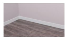
Clean any dried adhesive with denatured alcohol and a clean white rag, follow all manufacturers' precautions when using these type of products. Install Millwork or cove base or quarter round to complete the installation.
