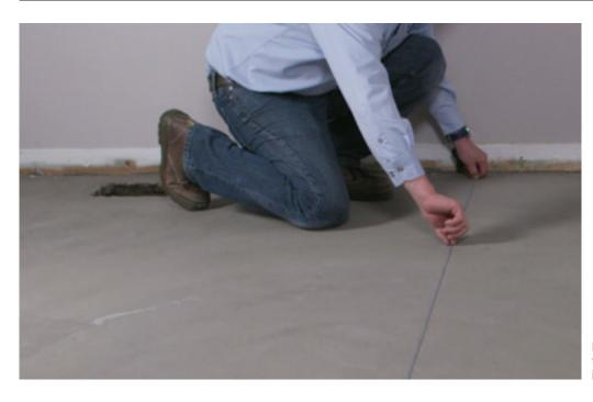
Establish a control line prior to adhesive application and installation.
