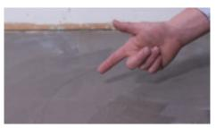
Allow the adhesive to go dry to the touch, a light touch with no transfer to the finger.
