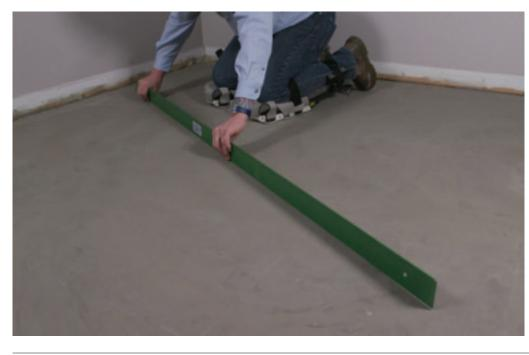
All substrates must be level within 1/8" in 8ft. This can be checked using a straight edge to identify any high and low spots. Any unevenness must be sanded down or filled with a cementitious patching compound.
