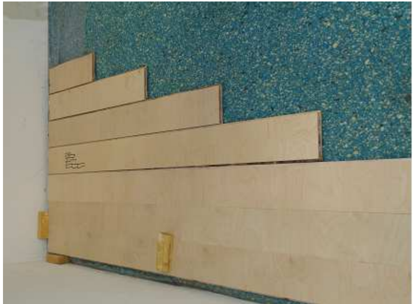
Cut the Lumaflex panels in order to obtain an homogeneous resistance Before assembling (the 3 first strips on this photograph)
