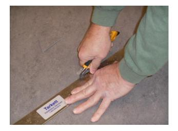
Making the third and final cut along the edge of the framing square. This ensures the damaged area cut out is just a little smaller than the insert to achieve a tight fit.
