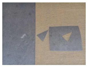
Make a third connecting cut to create the desired shape for the custom insert. The shape can be a triangle or diamond. Do not make a square insert as this will cause the final repair to be more noticeable. Determine the most common flow of traffic within the space. The seams should fall at an angle to the direction of the line of sight. Never allow a seam to fall perpendicular to the most prevalent line of sight.
