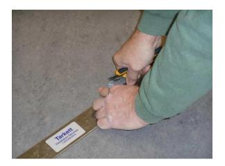
Lay the straight edge against the insert to help hold it in place. Carefully following the edge of the insert with a sharp utility knife, trace cut the flooring keeping the blade perpendicular to the flooring.
