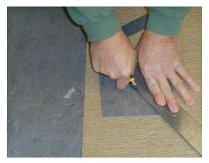
knife blade perpendicular to the flooring. Turn the straightedge and make a second cut while holding the knife perpendicular to the flooring. Be sure that the second cut connects to the first.
