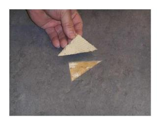
Using the recommended adhesive and trowel apply adhesive to the back of the insert.
