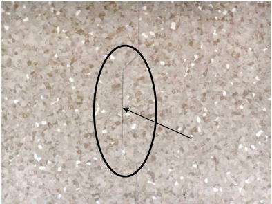
Using a recess scriber cut windows along the edge of the seam. At a minimum, one window should be made at each end of the sheet. After cutting the window, establish cross reference points on the top of both pieces.
