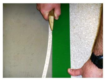
Remove a minimum of 1/2" from the factory edge of the first sheet. When utilizing a knife and straight edge be sure to hold the knife perpendicular to the floor.
