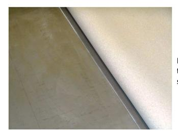
Fold the sheet back and use a white chalk line to establish a reference point onto the substrate.
