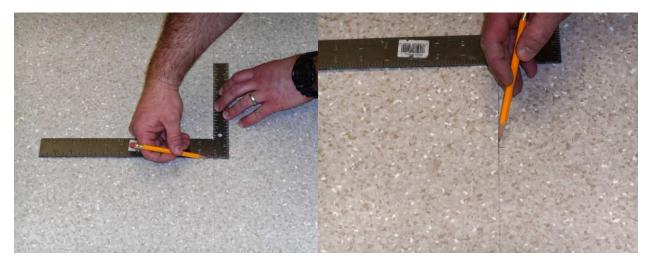
Using a pencil and small square establish reference points onto the top of both sheets. One mark should be placed perpendicular to the seam and another should follow the edge of the overlapping sheet.
