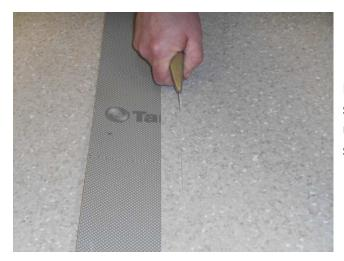
Place a piece of scrap material under the second sheet when cutting the seam. Utilize a utility knife with a sharp blade to cut along the scribe mark.
