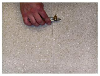
After applying adhesive following the steps outlined above, lay the second sheet into the adhesive and roll the sheet in both directions with a 100-lb 3 section roller. Be careful to keep the roller approximately 3" from the seam. Using a recess scriber, scribe the second sheet. The recess scriber should be preset to the desired width of the seam (no greater than 1/64" for heat welded seams).
