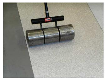
After laying the sheet into the adhesive, roll the floor in both directions using a 100 pound three-section roller.
