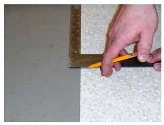
Establish cross-reference points onto the substrate and the top of the sheet.
