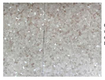
Clean any excess adhesive with a clean white cloth, dampened with water, before it dries. Erase all reference marks. Use to Denatured Alcohol to clean.
