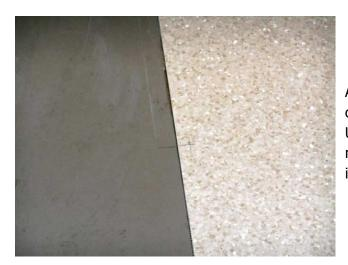
After the adhesive is allowed the appropriate open time, lay the sheet into the adhesive. Use the previously established reference marks to help position the sheet during installation.
