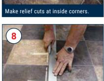
Place pieces of masking tape over seam edge to prevent movement. Using a sharp utility knife, double-cut through both pieces of flooring.
