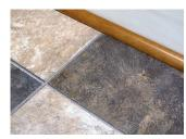
15. Install base board, quarter round or cove base to cover gap at perimeter. Nail into wall, not into the floor
