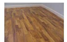
Continue until entire room is complete. Use of T-molding is required for rooms over 40'. Remove spacers and install matching quarter round and moldings.
