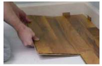
11. Install first plank of second row by inserting tongue side of plank at a low angle into groove side of previous row. Rotate plank downward until flat. Do not use tapping block to install long side of planks.
