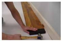
6. Using hammer and tapping block, gently tap along the groove side to engage each plank in first row. Tap in center of block. Continue in this manner to complete first row.
