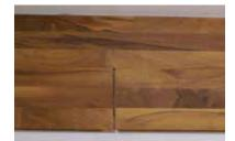
Slide plank toward previous plank. Position approximately 1/4" away from previous plank.
