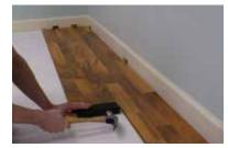
14. Using a hammer and tapping block, gently tap along the groove side to engage planks. Tap center of block.
