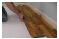
12. Install second plank by inserting the long side tongue at a low angle into groove side of previous row. Always stagger end joints from row to row a minimum of 12" (30.4cm).
