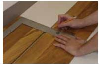
7. Measure and cut last plank in the first row. Allow for 5/16" spacer. Use a pull bar to engage last plank.
