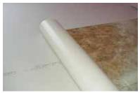
3. Install foam underlayment (Except Malibu and Worthington). When installing over concrete, install an approved vapor retarder prior to installing foam underlayment.
