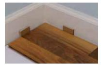
5. Place 5/16" spacers between wall and flooring. Align remaining planks in first row.
