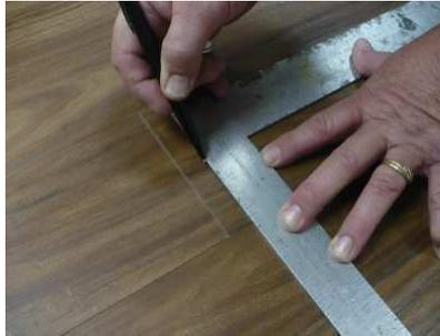
2. Using a straight edge and sharp utility knife cut completely through the plank along the lines. Using a hot air gun to warm the plank will make it easier to cut through the plank. Remove the center of the damaged plank.
