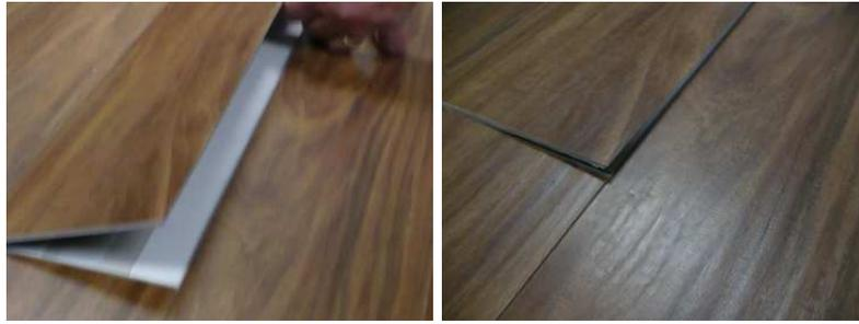
8. Wipe off any excess glue with a damp cloth. Roll seam edges with a hand roller to ensure proper contact with floating seam tape. Insure that all edges of plank are flush with the surface of adjoining planks. If necessary, place a smooth piece of plywood over the plank and apply weight until glue has dried.
