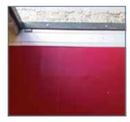
Aluminium one-piece transition strip used to join the sport flooring to surrounding floorings. Reinforced for heavy loading and striated for better grip. 4 different sizes to match various thickness differences. To be screwed.
